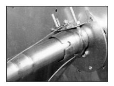
**P 9.** Place star lock washer [Y] over threaded stud above pulley, then add chimney cap [18] and fasten in place using 10-24 keps nut [21].
